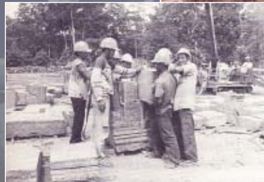
Reassembling of Stone Blocks
